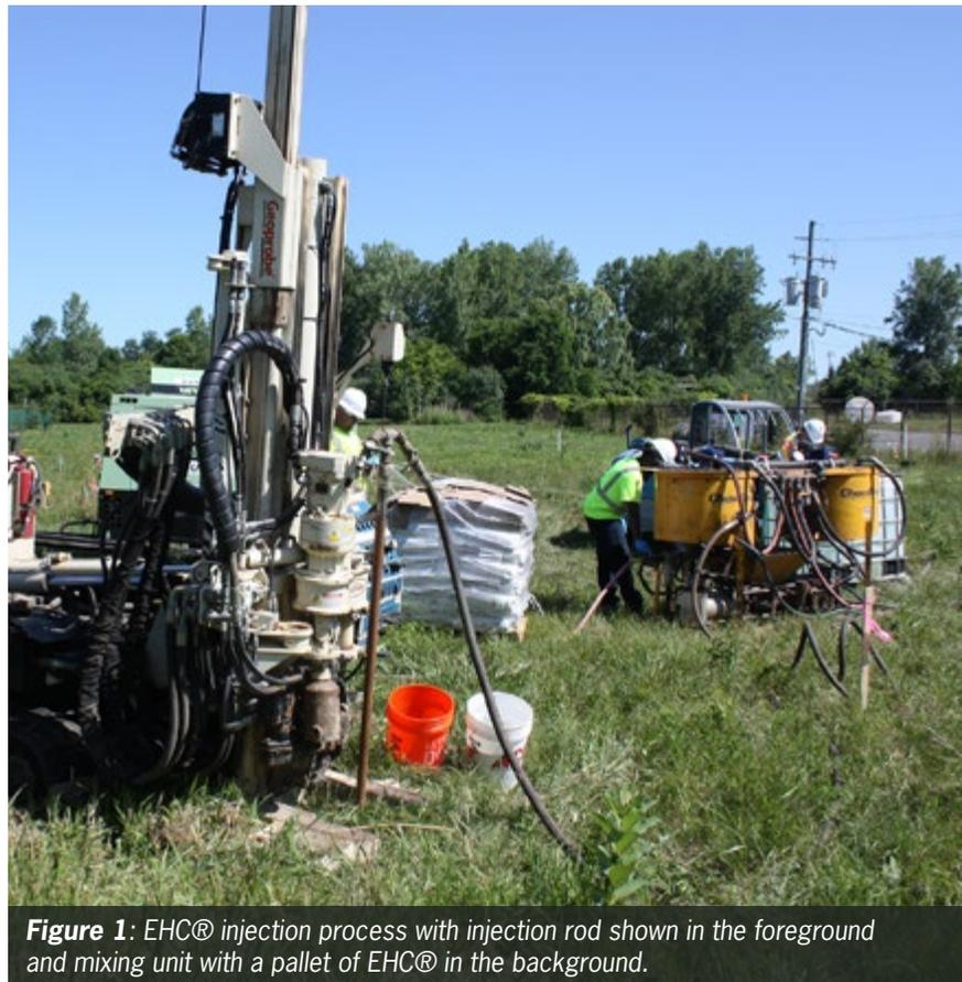
**Figure 1:** EHC® injection process with injection rod shown in the foreground and mixing unit with a pallet of EHC® in the background.
